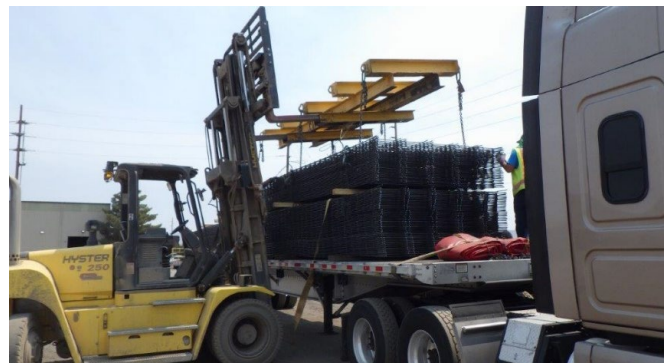
Figure 47: Forklift loading of WWR bundles onto truck
