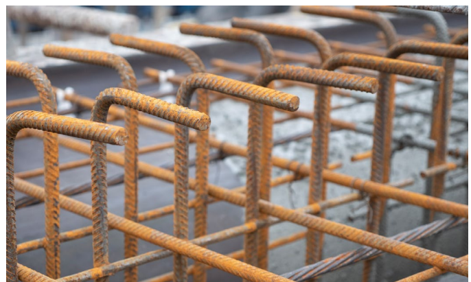
Figure 39: WWR mat used in the stem of a precast prestressed girder, showing bent terminations of stem reinforcement positioned to extend into a subsequently cast-in-place bridge deck.
