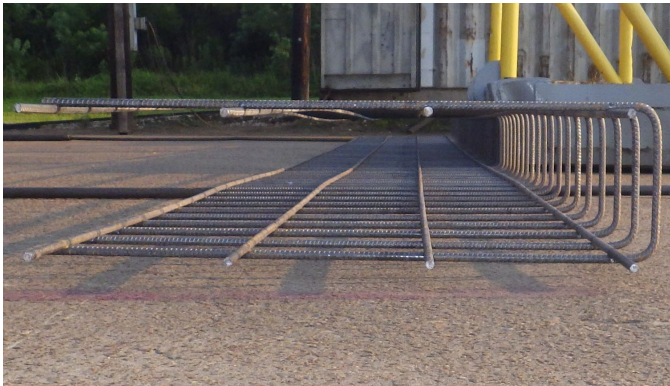
Figure 36: A down-the-line view of a bent WWR mat, shaped to suit a U-cage for use in a barrier rail.
