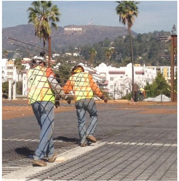
Figure 54: This project contained two distinct WWR usages: first, as a reinforcement for the topping slab over a structure constructed of precast double-tees (the mats can be seen staged on top of the double tees), and second as a reinforcement for a two-way mild steel reinforced elevated slab system (a unidirectional mat is being carried by the workers in the foreground, showing structural wires in one direction and non-structural holding wires in the transverse direction).
