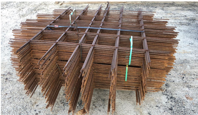
Figure 13: WWR mat bundle showing a configuration intended for a circular slab application
