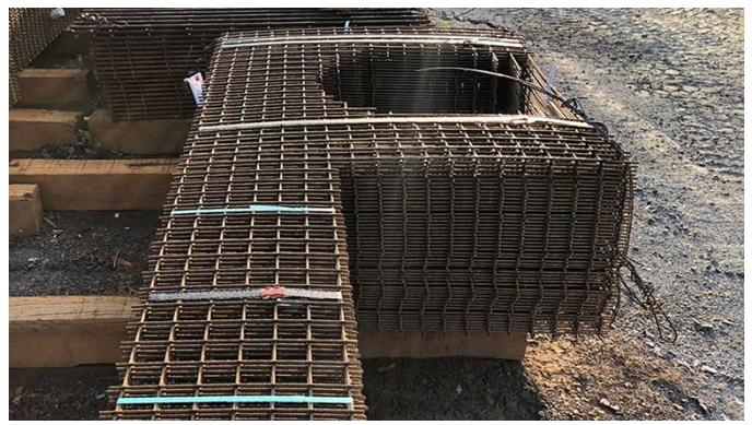
Figure 16: WWR mat bundle showing a configuration for use in a precast concrete element.
