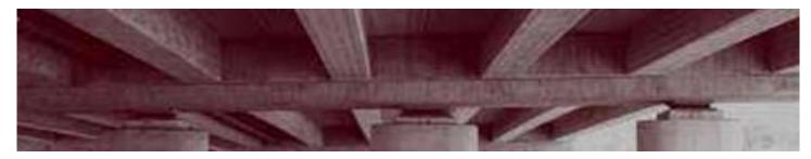
Cast-in-place pan joist slabs can provide economical concrete roof and floor construction. They are cast above reusable metal pans, foam panels, fiberglass or plastic pans, concrete or clay tiles, or other forms. Reusable pans are most frequently used. The ribs may run in one or two directions. This slab construction is generally known as "oneway pan joists" or "two-way pan joists."
