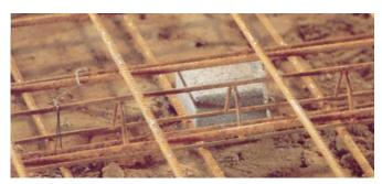
Place supports 2-3 feet apart for proper positioning of welded wire reinforcement during concrete placing. Concrete block, wire or plastic supports to hold reinforcement. These units are economical and effective.
