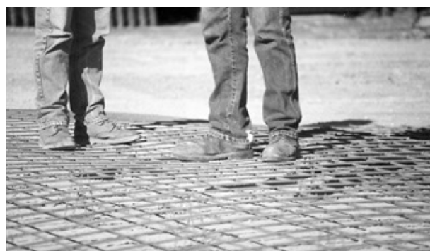
Figure 9.2. Welded wire is supported on steel wire chairs. Note stiffness of WWR.
