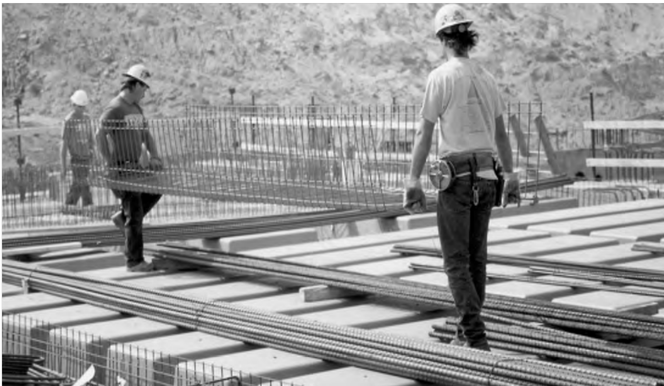
Figure 1.2. Placing a shear cage of welded wire reinforcement in a concrete girder for a sports stadium.
