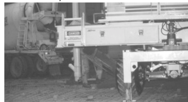
Figure 9.4. Laser screeds can ride over supported WWR. Maintain proper positioning when WWR is displaced.
