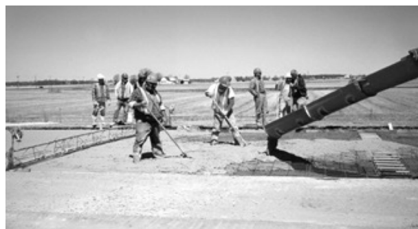
Figure 9.3. Welded wire used in repairing the Ohio Turnpike.
