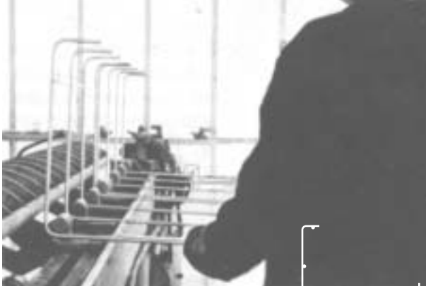
3RD BEND: Sheet has been advanced into machine and now another 90° bend has been made.
