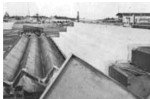
Form and completed riser
