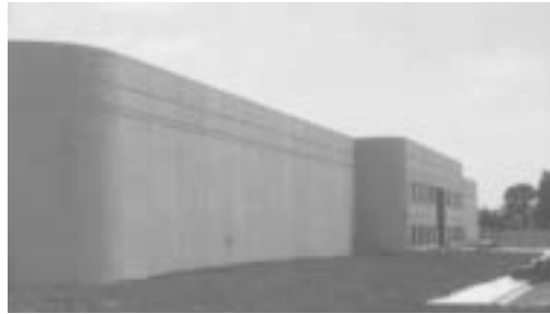
Flat and curved tilt-up wall panels make up the facade of this Ohio project
