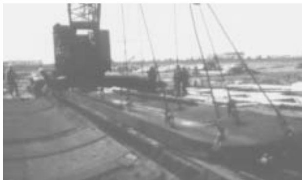
Large panel lift about to begin.
