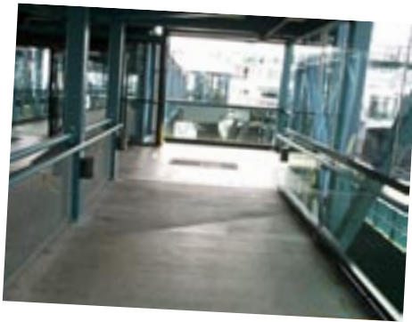
Pedestrian walkway, Bremerton Ferry Terminal, Washington State Ferries
