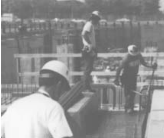
High strength WWR shear reinforcement allows excellent control of concrete cover and is very cost effective.
