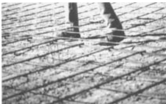
More cost effectiveness and easier placing can be achieved with step-through styles of WWR (12x12 and larger).
